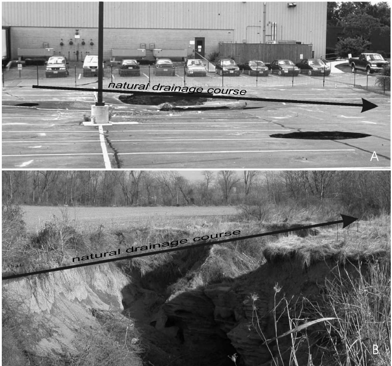
Figure 8. Examples of drainage lowlands acting as sites of sinkhole activity. (A) Parking lot built in the Ceresville Member of the Grove Formation in the northeast City of Frederick collapsed along the prehistoric drainage area. (B) Coalescing sinkholes in the Lime Kiln Member of the Frederick Formation along the drainage lowland in the southeast City of Frederick.
